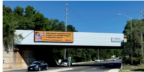
Bayview overpass before...and after
